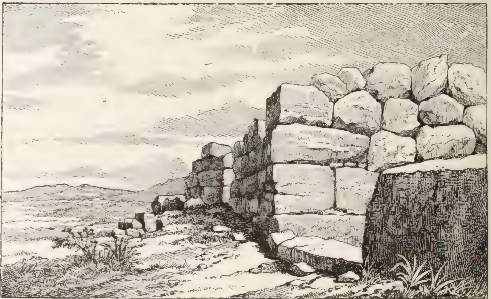
FIG. 71.—Tiryns: section of wall through the middle of the eastern face.
